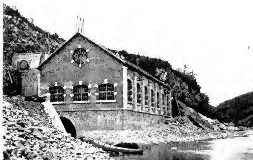
FIG. 2.—VIEW OF EXTERIOR OF POWER HOUSE.
